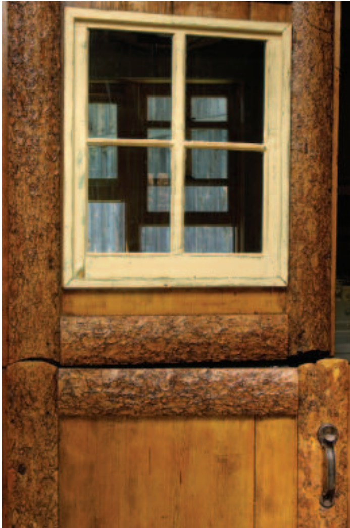
This Dutch door, with its four-paned window and split-lodgepole logs, was originally an exterior door of the cabin. Today, it opens onto the laundry room.
